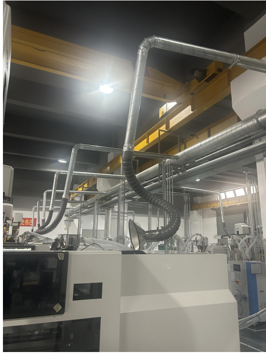
DA001 废气装置集气罩
